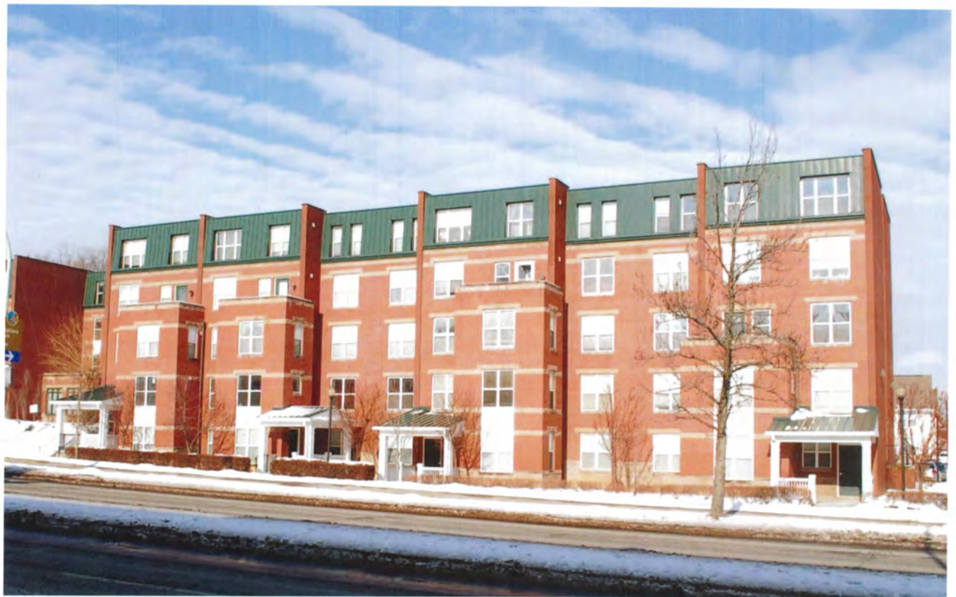
Image 1.2: Buildings are located across Penn Avenue from one another, but were once identical in terms of appearance. Façade alterations on the bottom building occurred c. 2005 Source: Justin Greenawalt
