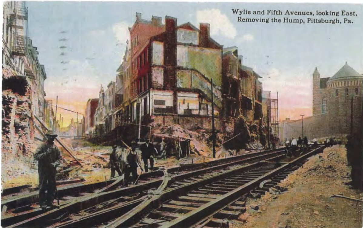
Image 2.4: A civic improvement effort known as the "Hump Removal" took place c. 1912 in Pittsburgh's Downtown. The "hump" was the remainder of the historical Grant's Hill which had made traversing Downtown's eastern portions difficult due to its steep grade. The removal of the "hump" served to remove some of the Downtown district's most dense building stock and provided the opportunity for the construction of such historically inspired buildings as the Union Arcade and William Penn Hotel. The building seen on the right is the F.J. Osterling addition of Richardson's Allegheny County Jail. Source: Postcard. Author's Personal Collection
