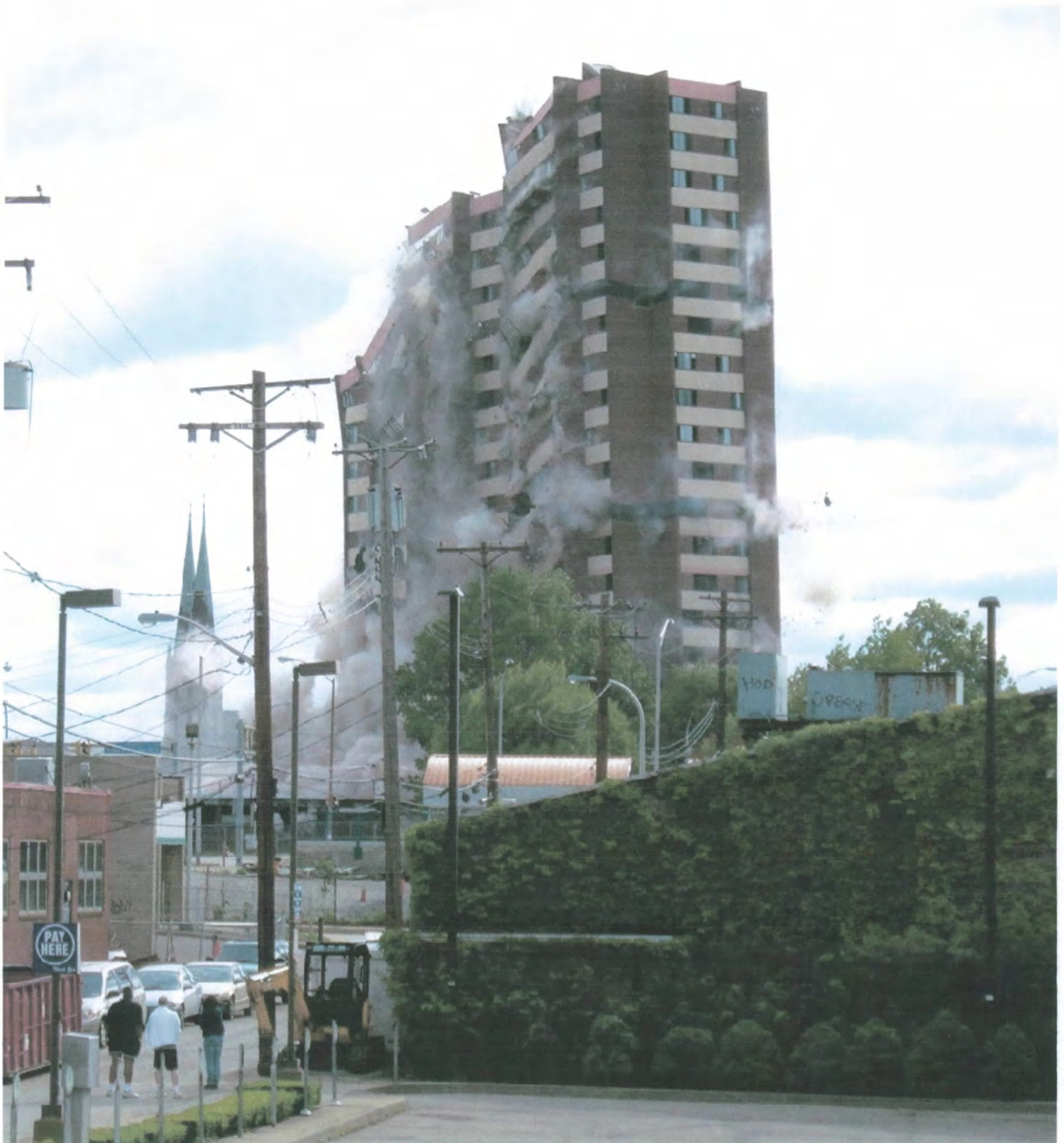
Image 6.9: Implosion of Penn Circle Apartments, May 2009
