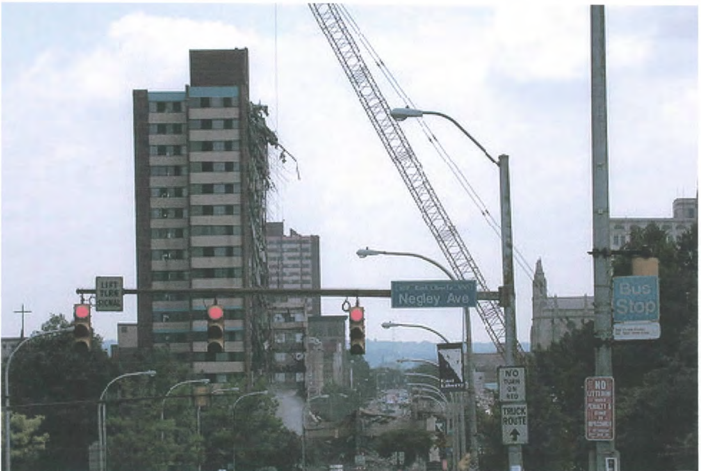
Image 6.8: Demolition of East Mall Apartments in 2005
