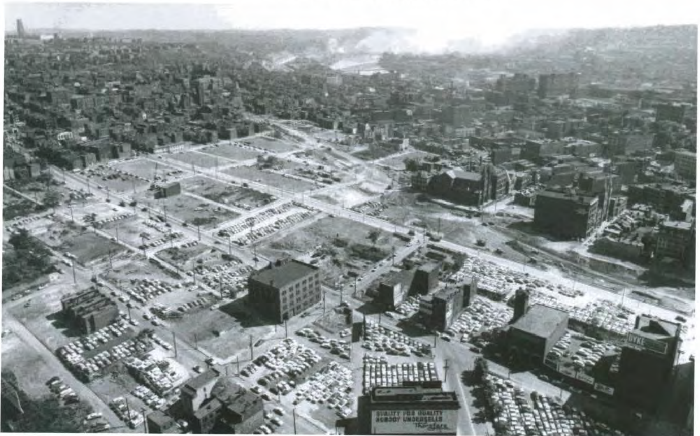
Image 3.9: Demolition of the Lower Hill district for construction of the Civic Arena, August 1957 Source: University of Pittsburgh Digital Archives: Historical Society of Western Pennsylvania
