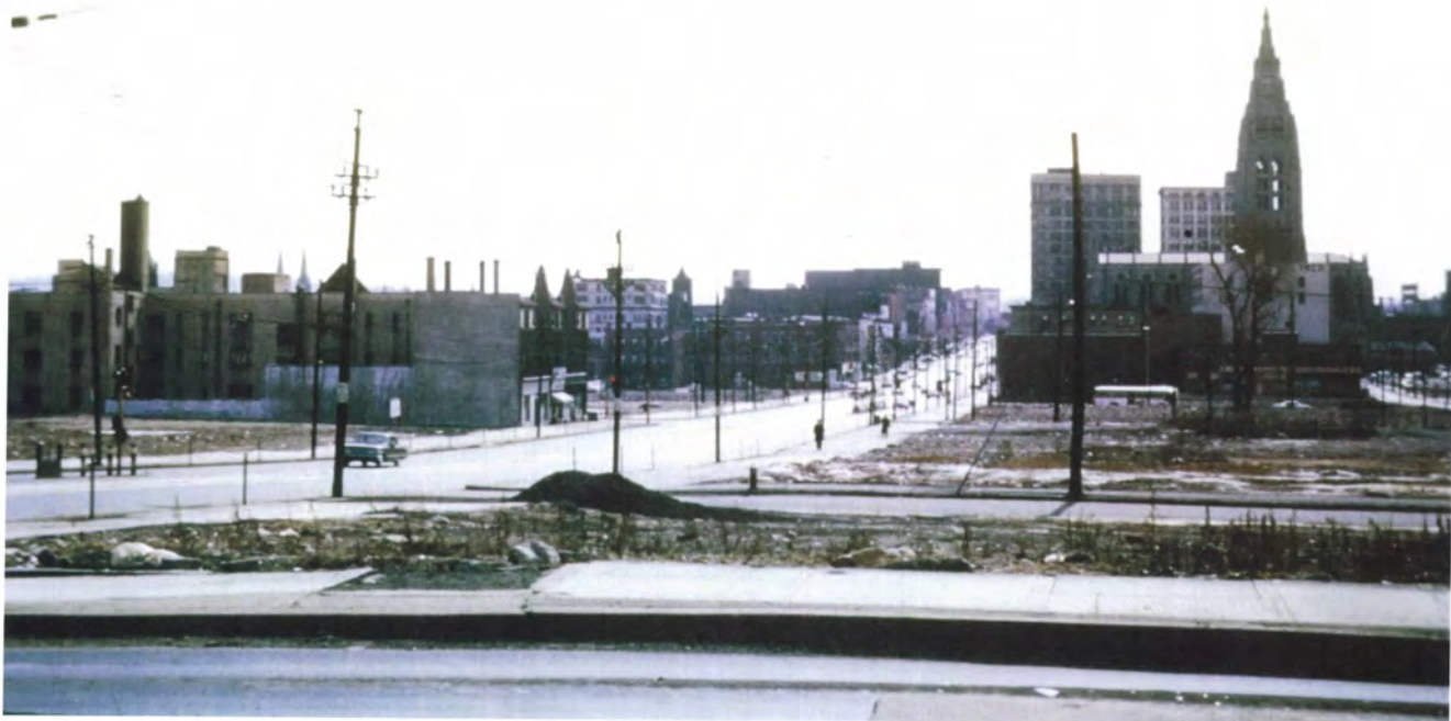
Image 5.17: Demolition for East Liberty Project. Penn Avenue at Euclid Street (Penn Circle West) Source: Pittsburgh History & Landmarks Foundation
